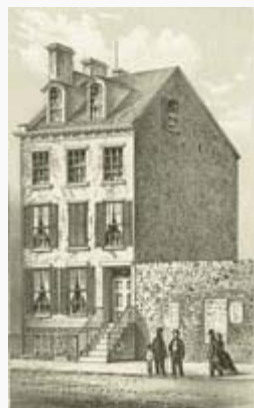
Pearl Street Station Exterior
