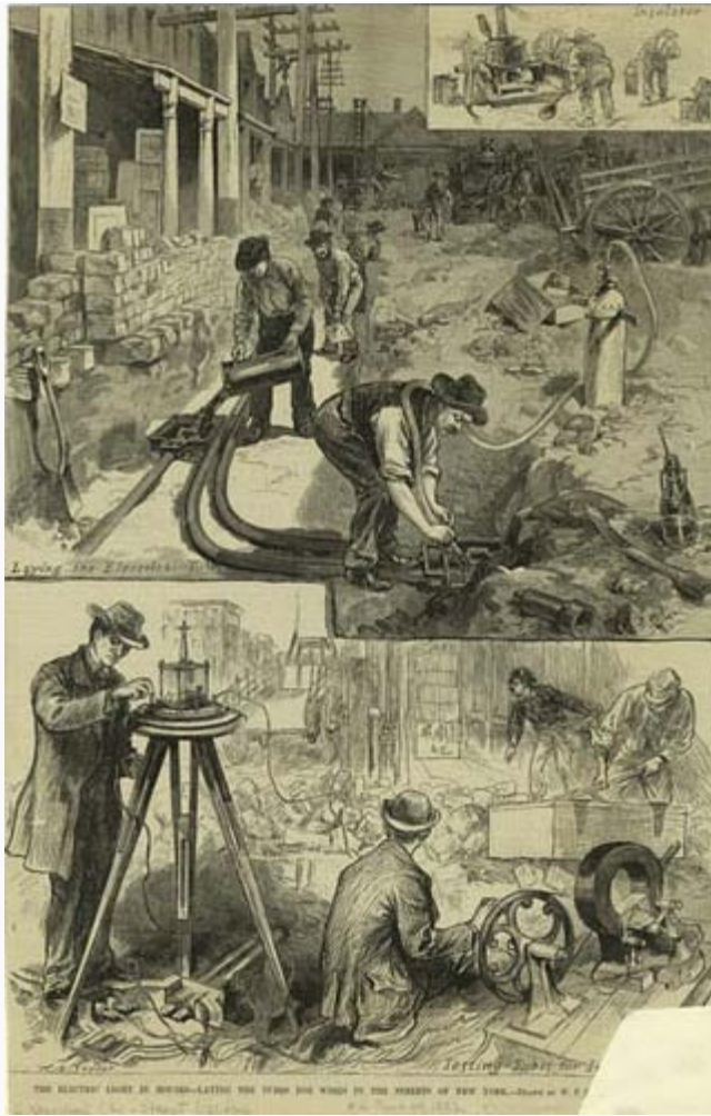
Pearl Street Station Laying Wiring
